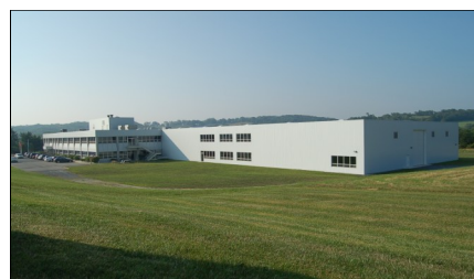
Verticon, Ltd. built this impressive facility for fellow Council of Industry member, Baser Swiss Lube, in Goshen, NY.
