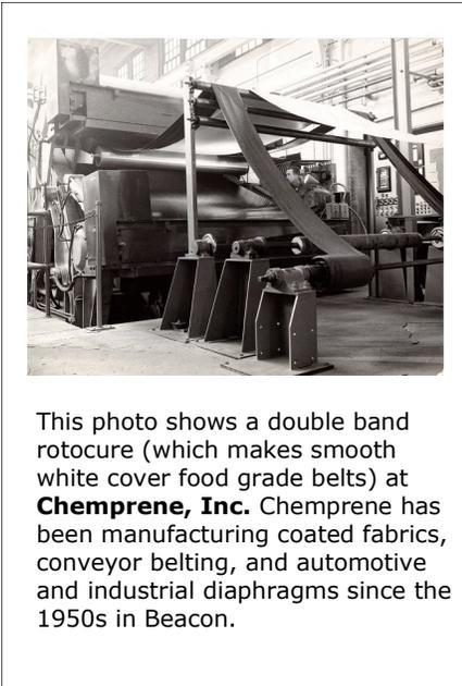
This photo shows a double band rotocure (which makes smooth white cover food grade belts) at **Chemprene, Inc.** Chemprene has been manufacturing coated fabrics, conveyor belting, and automotive and industrial diaphragms since the 1950s in Beacon.
