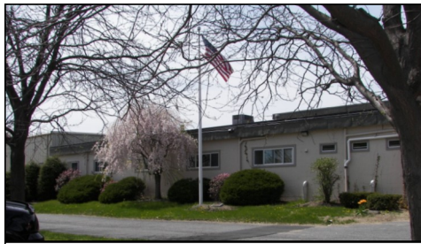
Viking Industries, Inc. facilities in New
